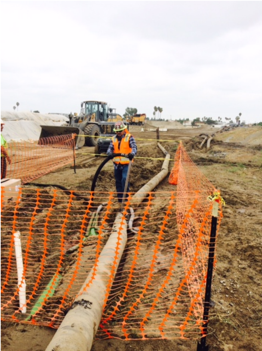
Photo 2: Vacuum truck recovering liquids from pipeline excavation.
