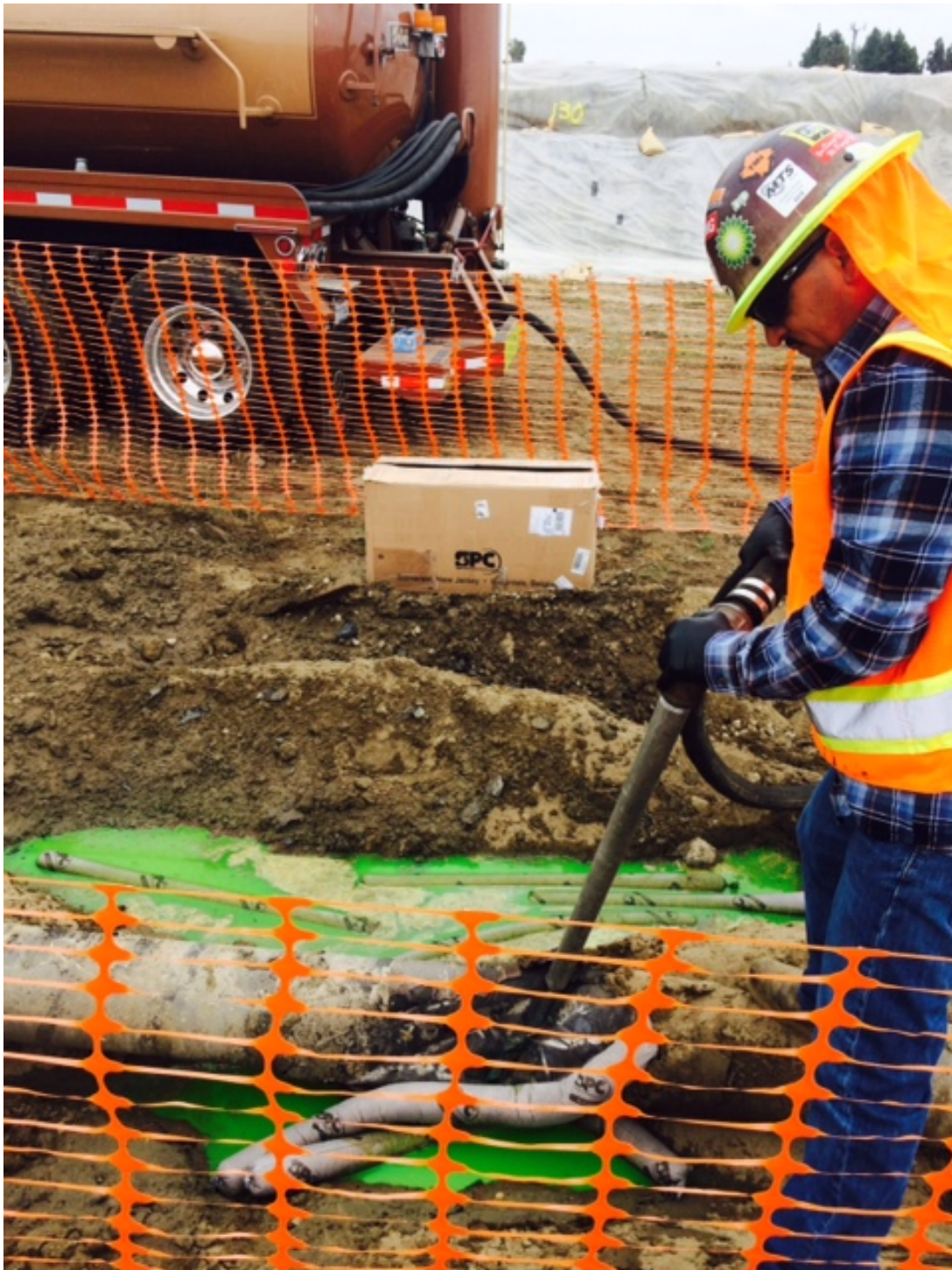
Photo 3: Vacuum truck recovering liquids from pipeline excavation.
